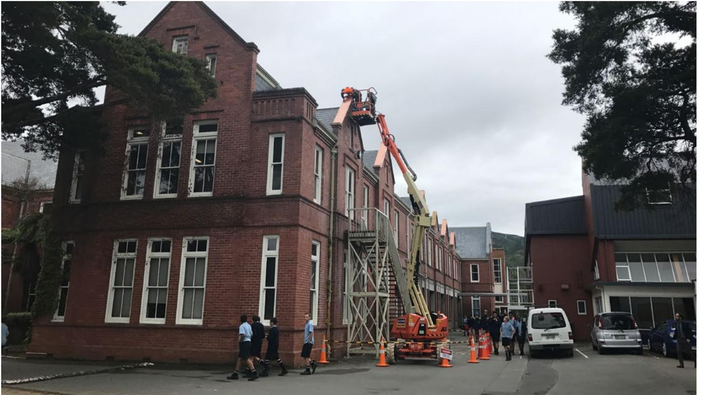
The completion of the strengthening of the parapets, with copper flashings.
